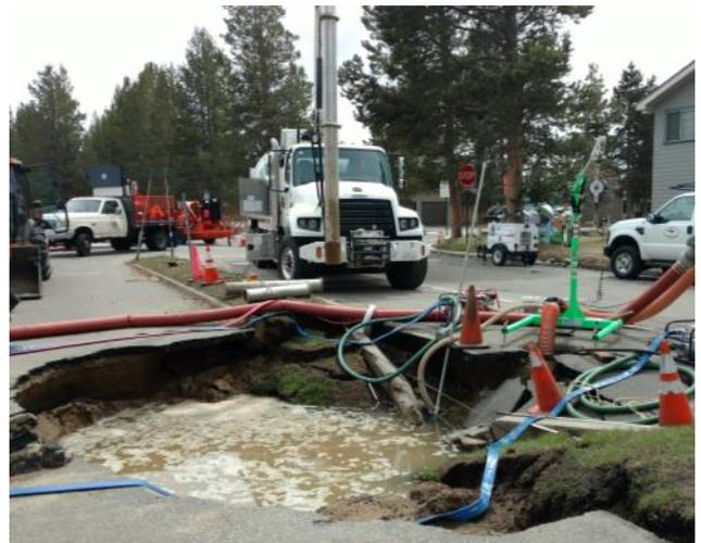
*A sinkhole formed on Tahoe Keys Blvd in 2017 due to the collapse of an old sewer pipe. Costly emergencies like these could become more common without increased investments.*
