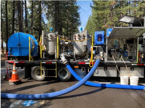
The flushing truck is attached to two fire hydrants. One hose pumps water into the water main at a high pressure and the other hose returns water to the truck to be filtered and tested before being pumped back into the water system. This process minimizes water loss.
