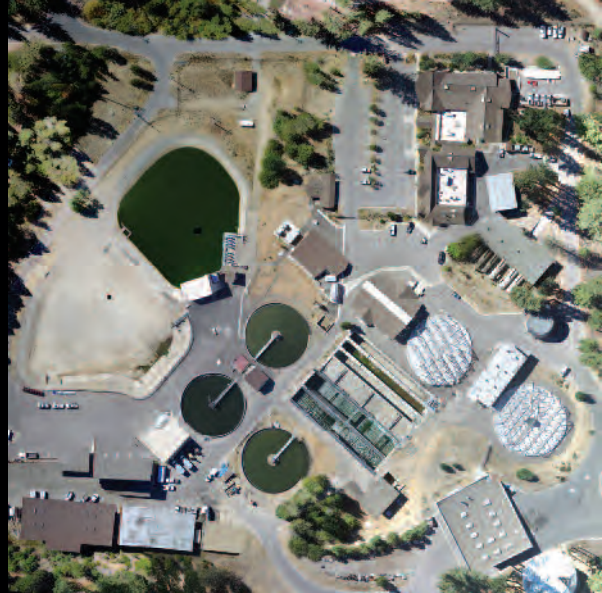
STPUD Wastewater Treatment Plant 2020
