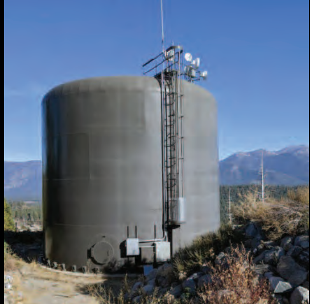
Angora Water Tank 2010
