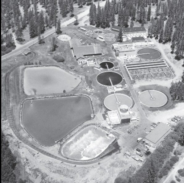
STPUD Wastewater Treatment Plant 1960s
