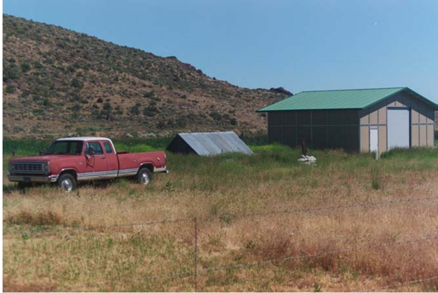
Figure 3. GW-04: Septic tank and leach field.
