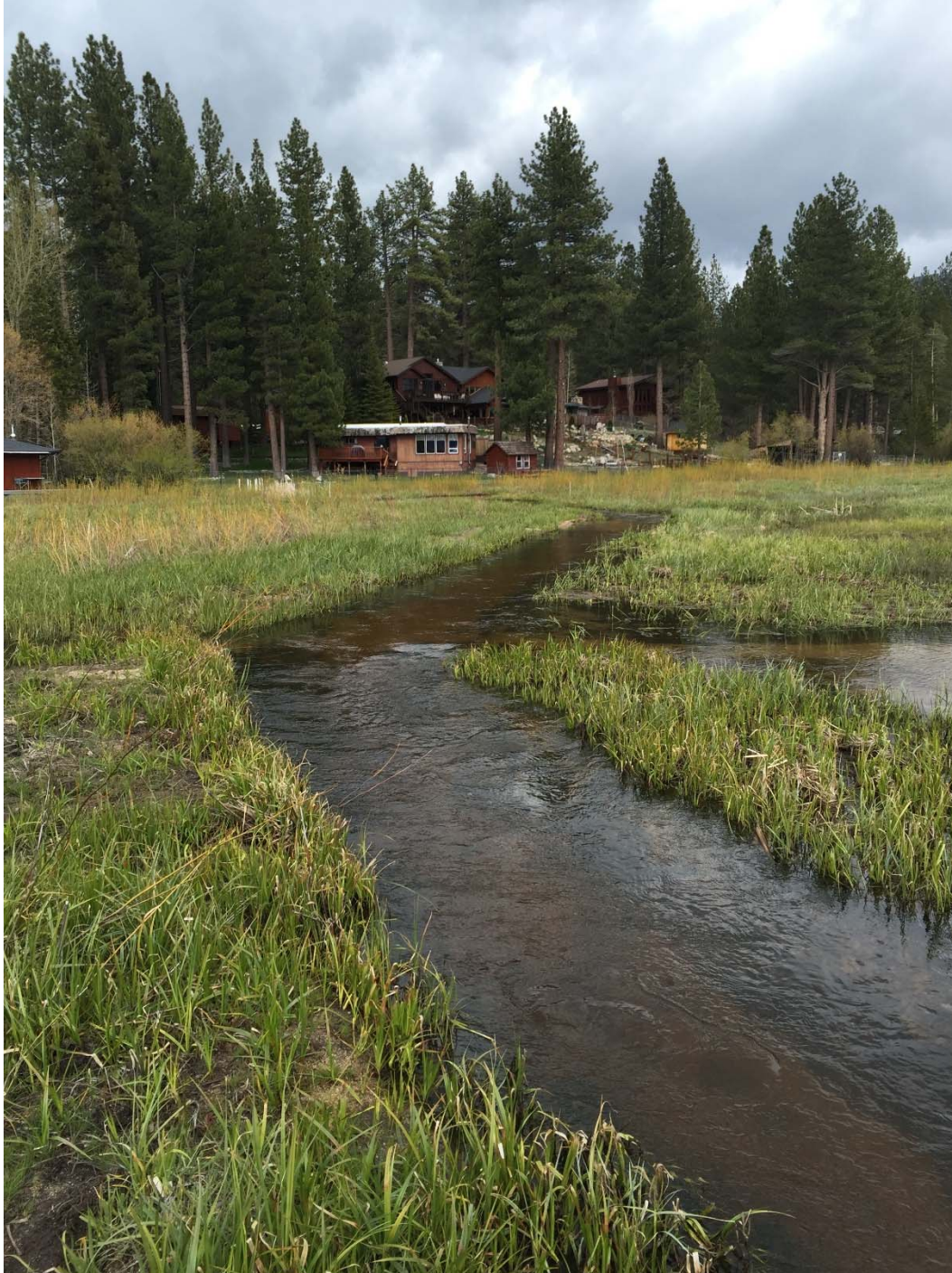
Photo 4. Pilot Channel 3 flow, about midway between head and outlet. Right overbank (left side of photo) revegetating after use for construction access and spreading of excavated material in 2015.
