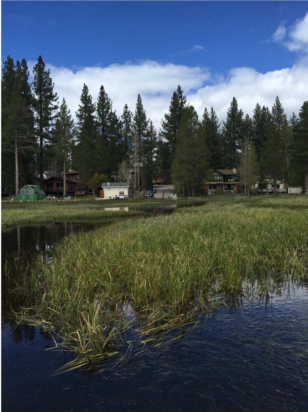
Photo 2. Near pilot channel return (in foreground) looking towards Bellevue PS. Overbank flow shallow, low velocity. PC return flow velocity about 2 fps (foreground).
