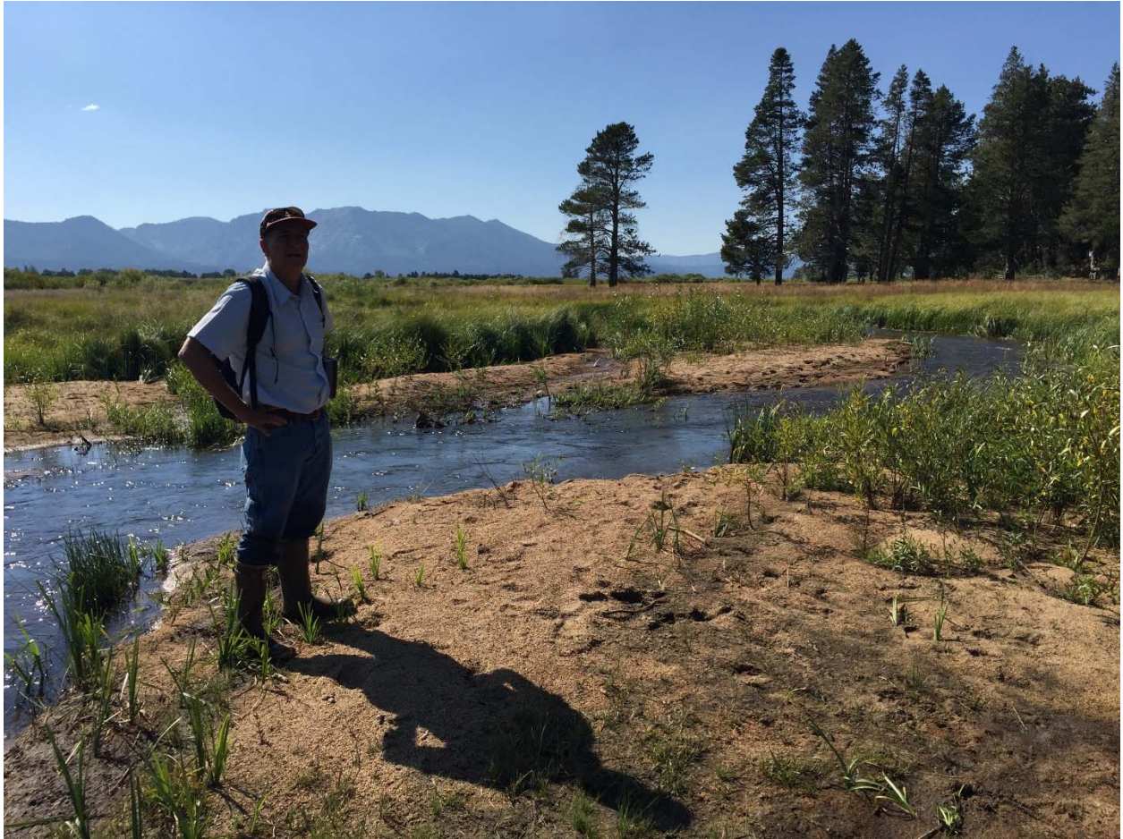
Photo 11. Deposition from overbank flow on pilot channels, approximately 100 feet upstream of outlet. Pilot channel flow at about 2 fps.
