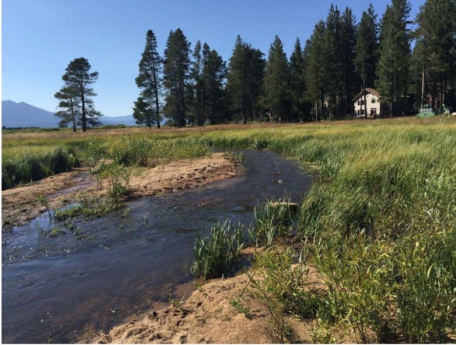
Figure 4-2. Pilot channel flow looking downstream approximately 100 feet upstream of confluence with Trout Creek showing overbank deposition of sand during high flows, 9 Aug 2016
