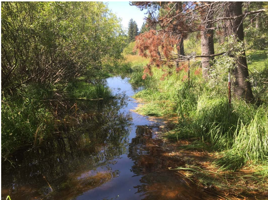
Figure 4-11. Inundation in District easement downstream of Manhole BV22, Aug 2016
