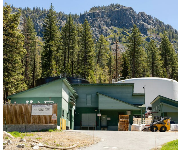
Luther Pass Pump Station
