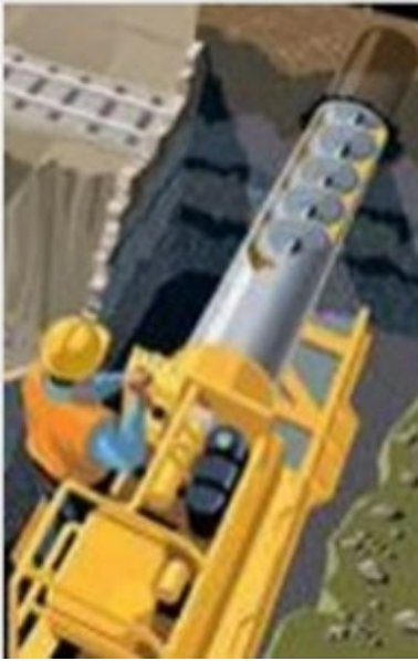
Figure 3B.2 Auger Boring
