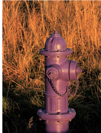
Urban Fire Protection
